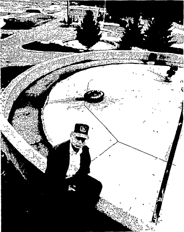
Fred Thalmann, superintendent of the joint Madison and Chatham sewer plant, sits outside the facility described as in need of repair
